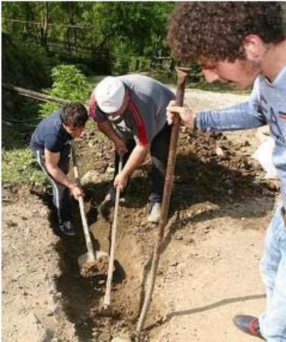
**Photo 2. Kvashta village, drainage channel under construction**
