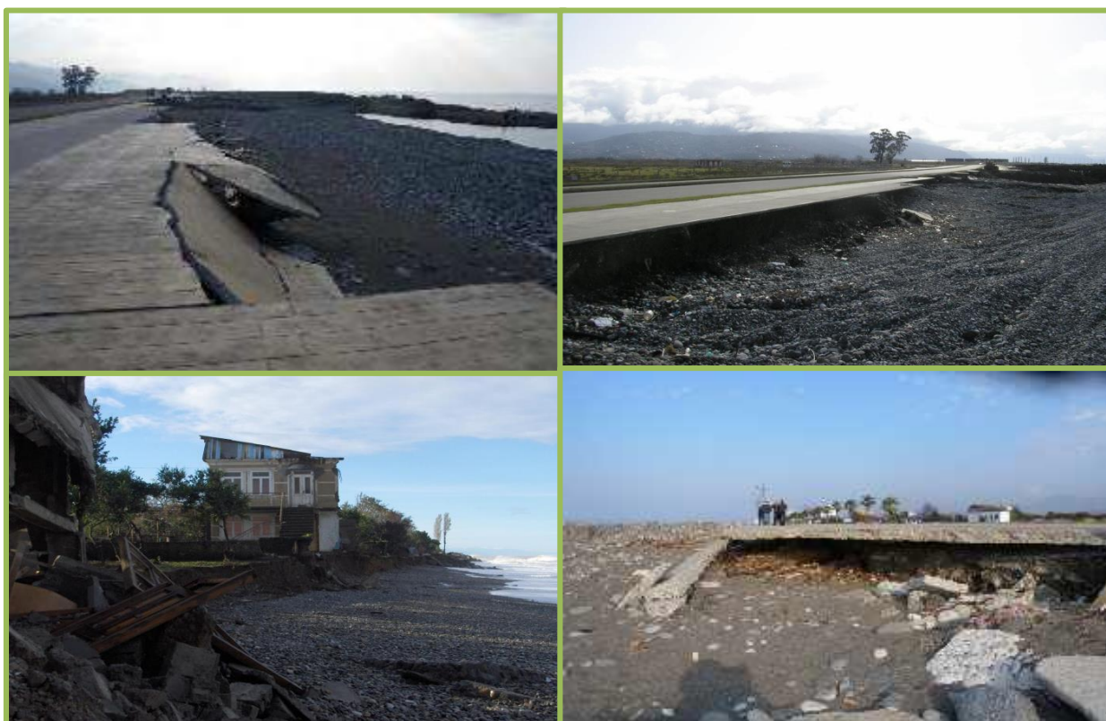
Fig. 3.18 Condition along the coastline with damaged infrastructure built recently 80
